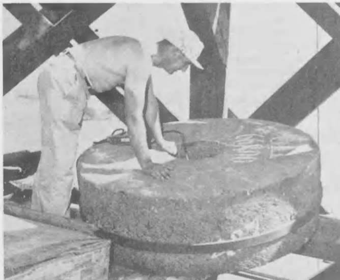
INSPECTING A grinding stone is J. Medendorp, one of four mill builders left in Holland, who came to Aruba to erect the mill. At right is a section of the wood gears which transmit power to grinding stones.
